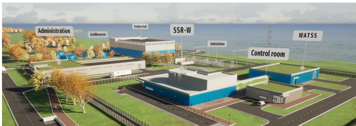
Figure 1 SSR-W plant layout including GridReserve® storage system (semi-buried tanks at the back)
