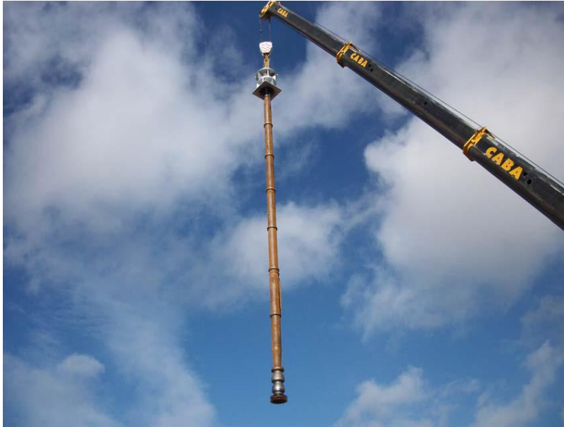
Figure 9 Flowserve molten salt pump 18CKXHF-2 prior to installation in tank [4]
