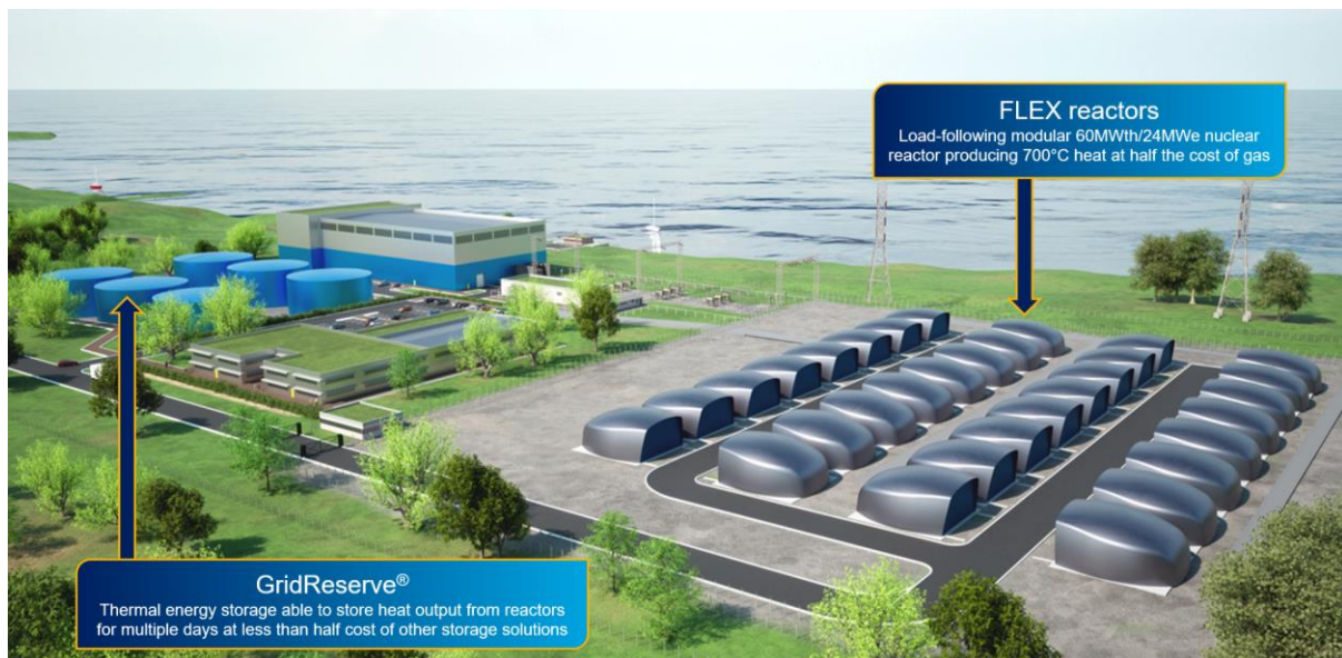
Figure 2: Artist's impression of a power station with a 32-module reactor array, GridReserve ® and turbine hall
