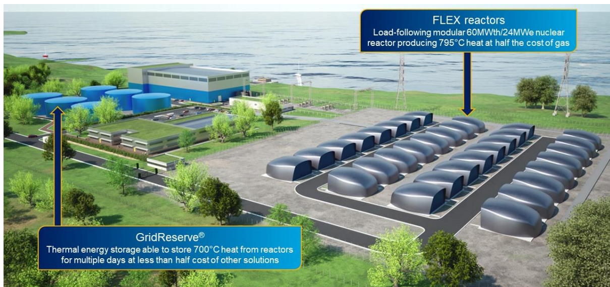
Figure 2: Artist's impression of a power station with a 32-module reactor array, GridReserve ® and turbine hall
